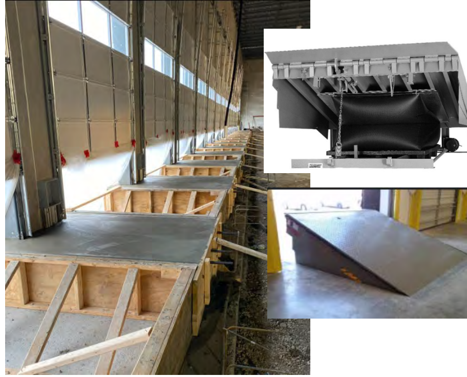
Dock pits prepped for levelers
